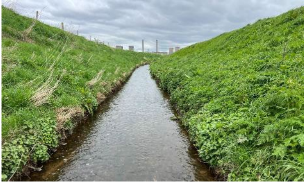
Photograph 7.3.17: Example of large drains, Catchwater Drain (other rivers and streams)
